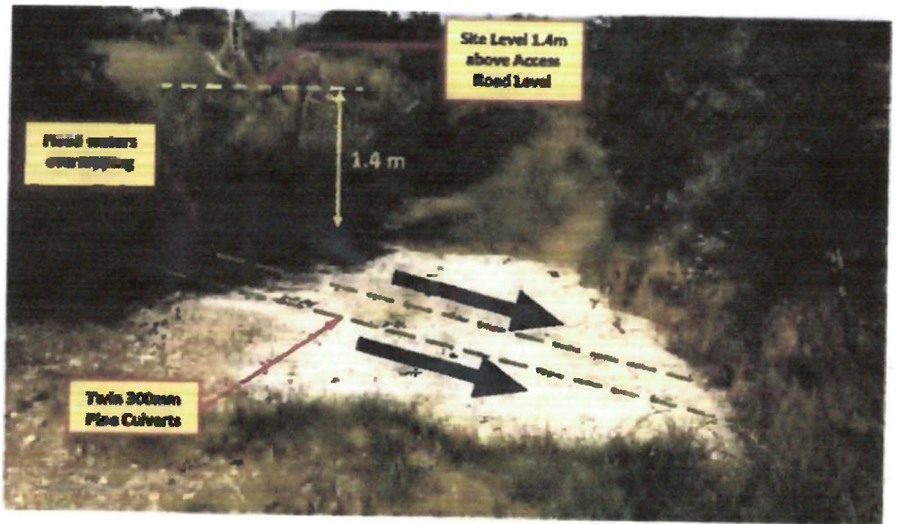
Figure 19 – Twin Culverts Overtopping Field Access Way
